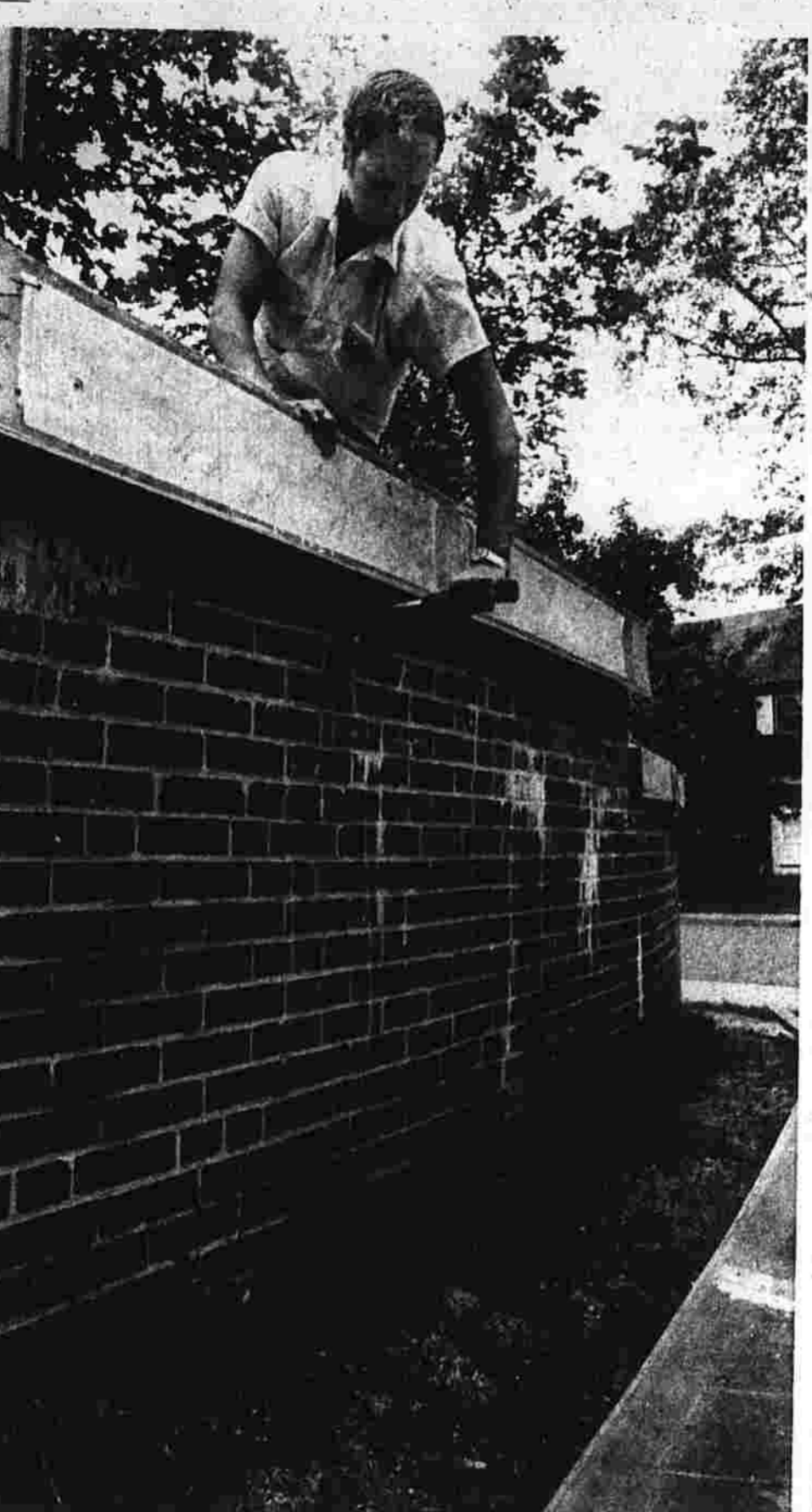
Repairing Retaining Wall
